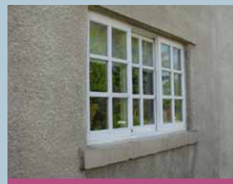
Traditional architectural details such as these Yorkshire horizontal sliding sash windows are important to the character and appearance of Barwick
