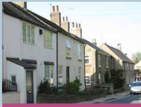
There is a variation in the finish of properties on Main Street. The most predominant finishes are exposed stone, or full render
