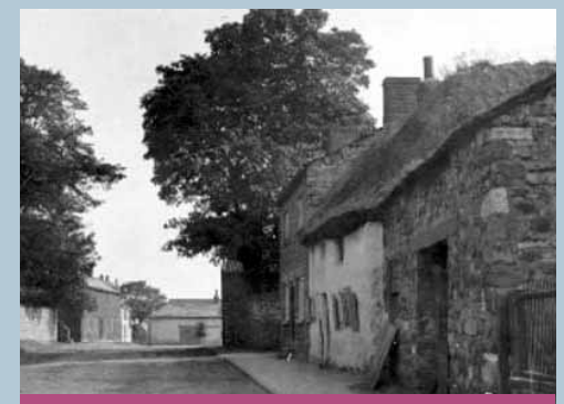
Historic photographs highlight many of the building characteristics which are still important today, such as variation of wall finish and domestic scale
