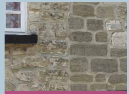
Coursed stone, of varying qualities, is the most dominant building material in the conservation area.
