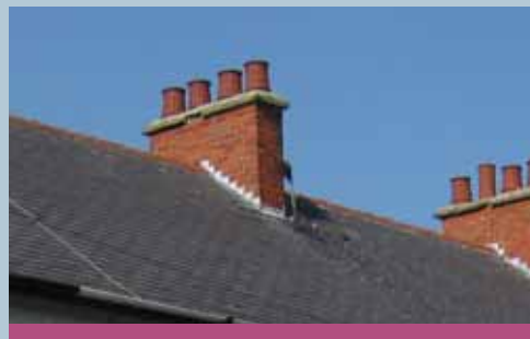
Traditional slate roofing materials are important to the roofscape of Barwick.
