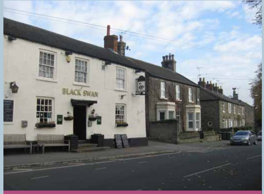
The back of pavement edge location of properties gives the conservation area an enclosed feel in some locations.
